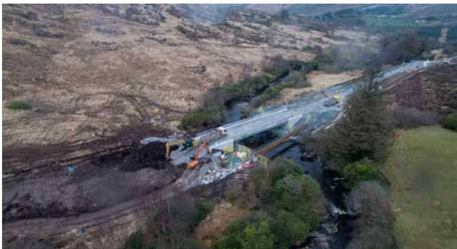
Access Bridge crossing the River Roughty
